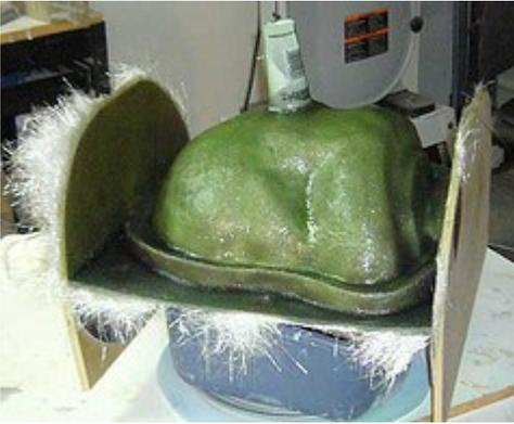
Here is a tip: If you wait until the resin gels (gets firm, but not completely hard) you can run a utility knife along the edge and trim a nice clean edge. If you wait until the fiberglass is completely hard, you will need to grind the edge with a belt sander to get a clean edge. GRINDING FIBERGLASS IS MISERABLE- AVOID AT ALL COSTS
